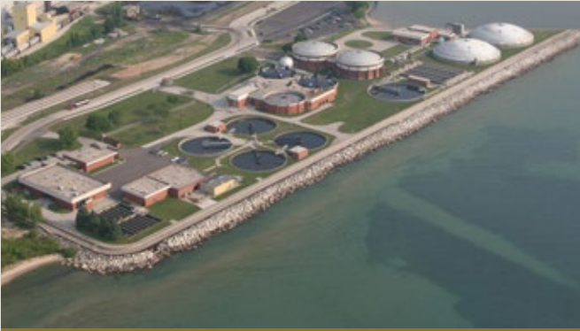
Aerial view of the Wastewater Treatment Facility
