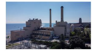
Boiler 8 ran successfully on 100% renewable densified fuel pellets this past year. Our second boiler, Boiler 9, is burning up to 40% pellets and that percentage is expected to rise. While we've been making this shift in our boilers, we've been concurrently working on increasing the supply of densified fuel pellets that MPU is able to secure.
